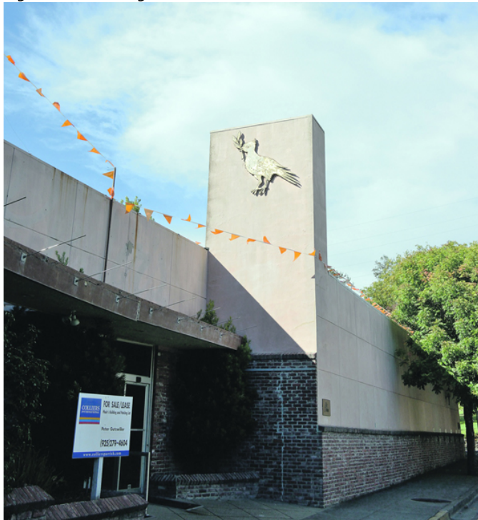
Phair building on Avenida de Orinda Photo Ohlen Alexander
