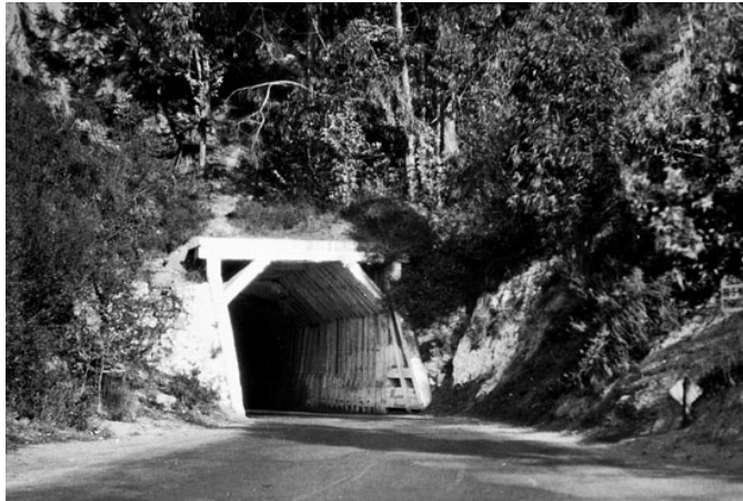
Kennedy Tunnel western entrance, 1924 Photos courtesy Lafayette Historical Society
