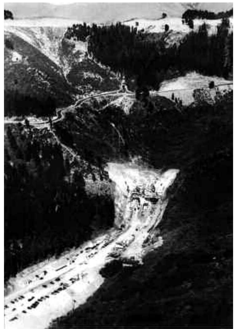
The Broadway Low Level Tunnel. “The first phase of construction involved clearing the hillside and grading (shown here on the Oakland side). The Kennedy Tunnel and the original roads leading to it are visible in the upper part of the photograph. The lower location of the new tunnel meant a shorter climb but a greater distance for construction workers to bore.”
