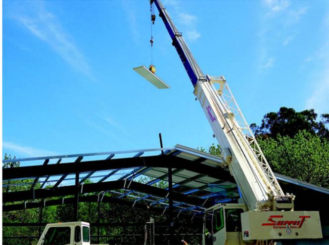
A crane uses powerful vacuum suction cups on an assembly to hoist roofing panels on the new Manzanita Room in Lafayette. Photo Cathy Tyson
