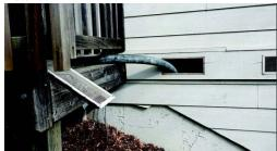
Concrete is delivered into the crawl space via the easiest route - in this case, a vent opening.
