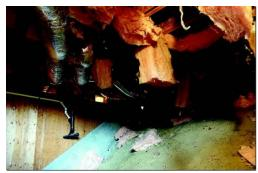
Rats may disturb the insulation from between the floor joists. After the slab cures insulation must be reinstalled.
