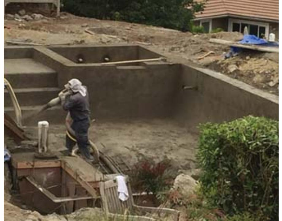
Gunite is sprayed over steel rebar forming the pool shape. Oversized first step is called a sun shelf.
