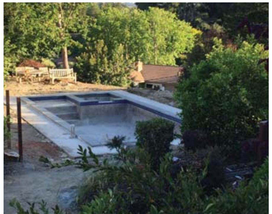
Decorative tile installed; Pennsylvania blue stone used as coping stone is mortared to the top of pool.
