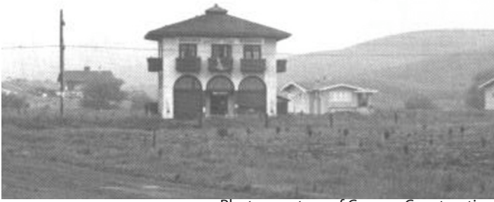
Photo courtesy of Canyon Construction
