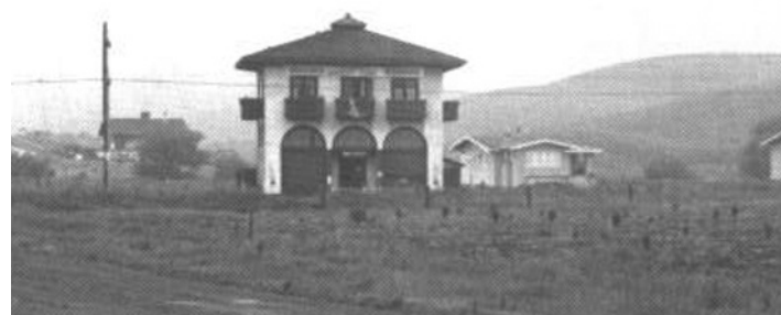
Photo courtesy of Canyon Construction
