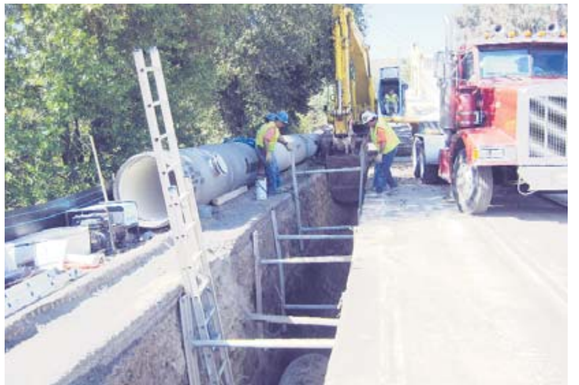
7-ton pipes are set in a 10 foot deep trench
