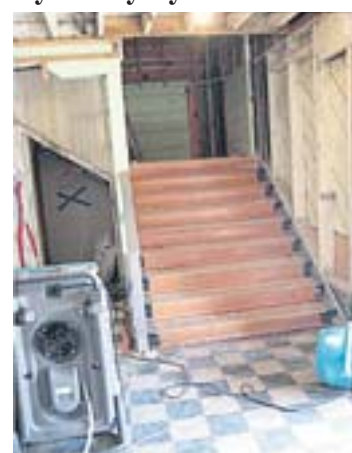
Lobby stairs Photo provided
