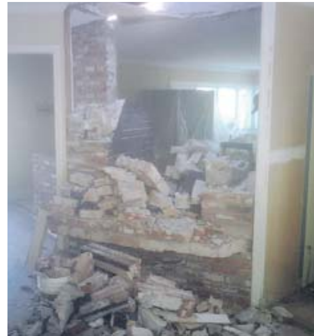
The Keough's old fireplace was demolished
