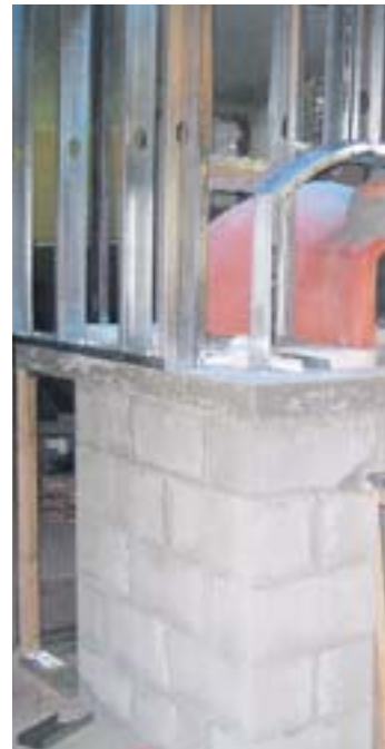
Building the pizza oven
