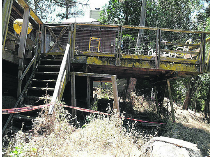
View of sagging back deck of vacant Ruth Court home Photo Cathy Tyson
