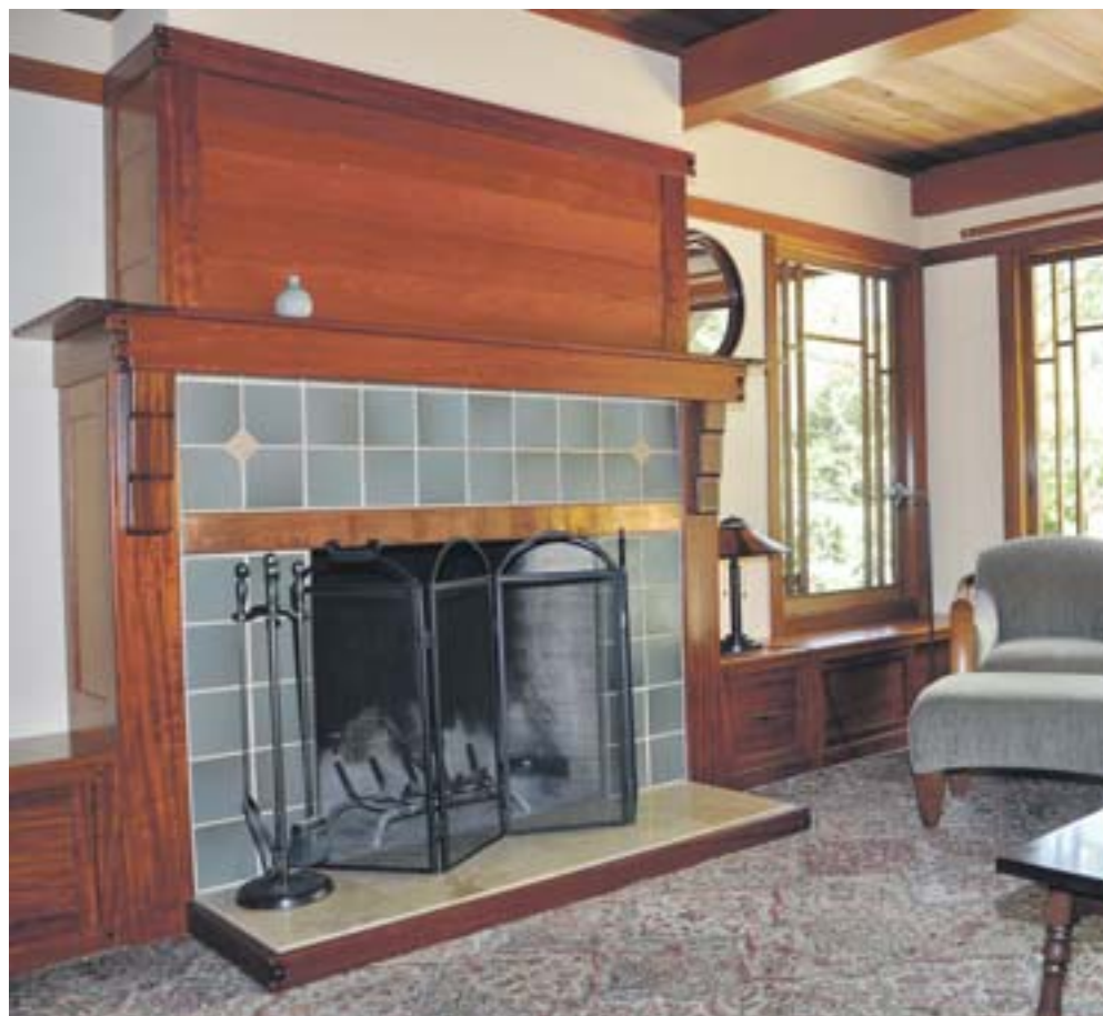
Steve Kauffman's fireplace, created in a combination of wood, tile, and copper
