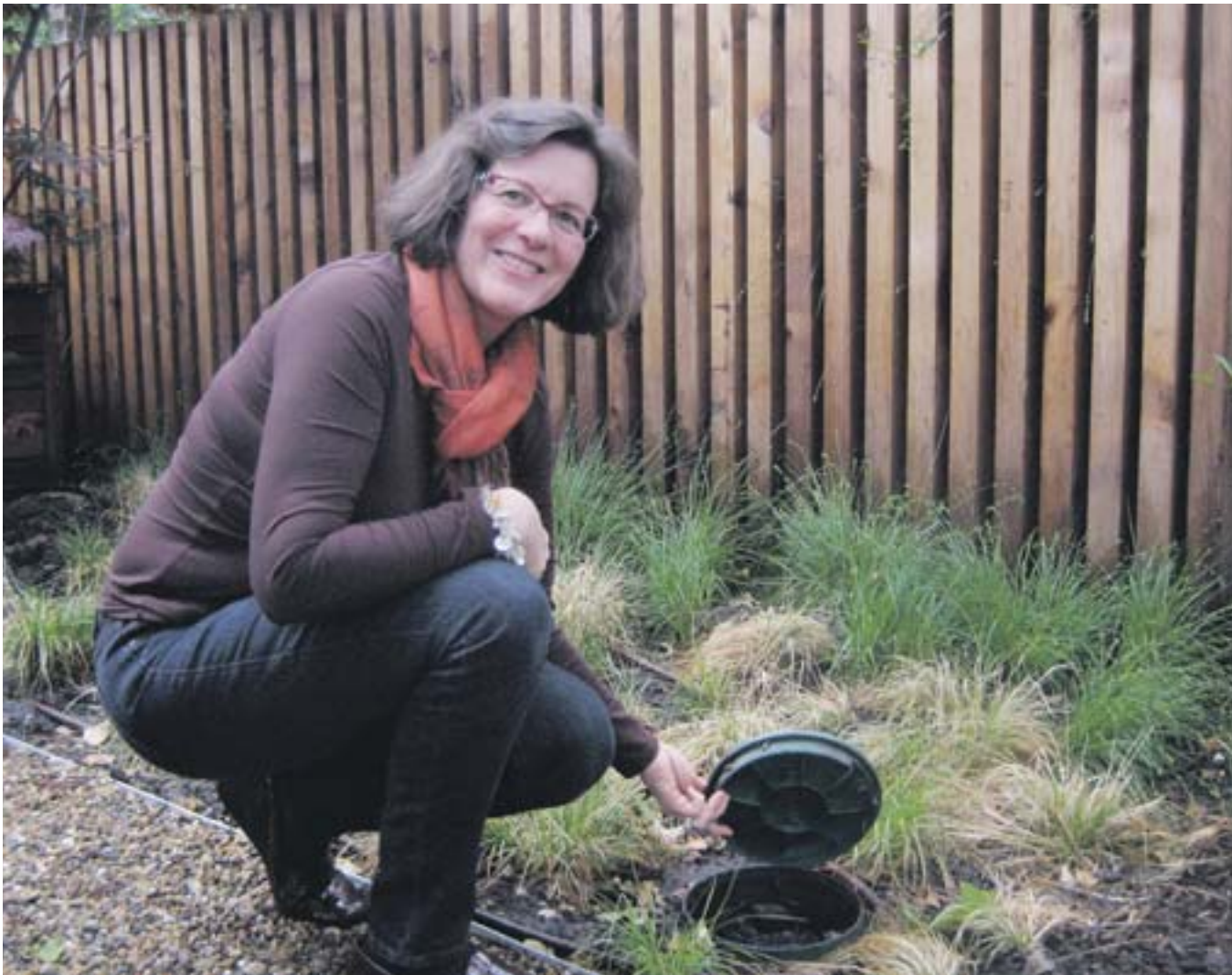
Gwenn Lennox shows the entrance to the gray-water collection tank.
