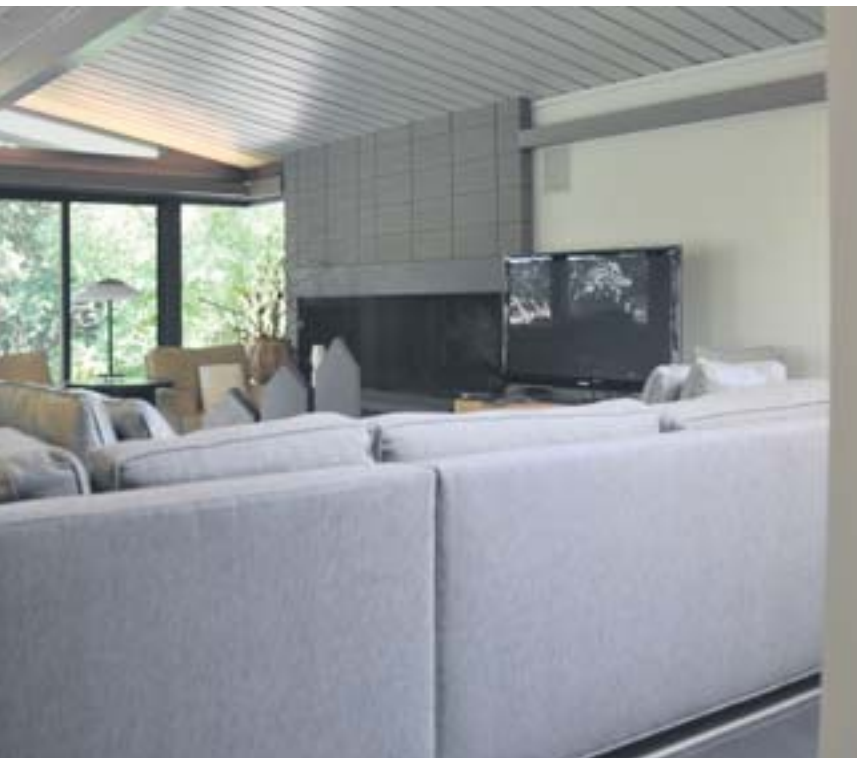
new cement cladding on existing fireplace.
