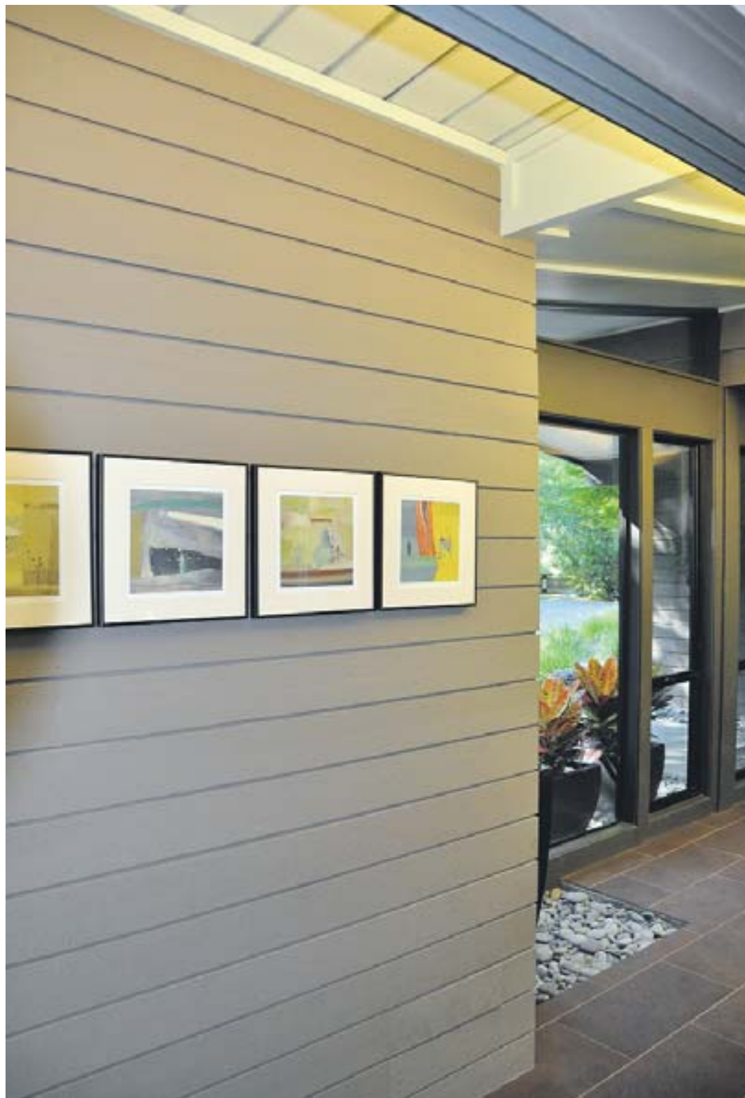
Re-purposed original decking was used as a wall treatment in the main hallway.
