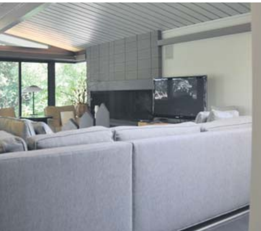
new cement cladding on existing fireplace.
