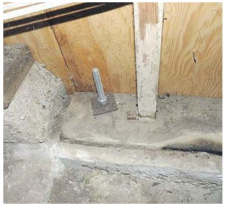
Retrofit anchor bolt with plate washer (on left) shown next to original anchor Photos Cathy Dausman bolt and small washer.
