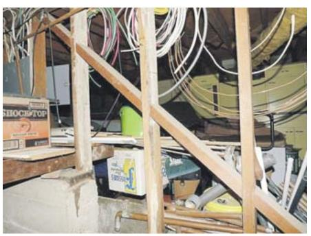
An example of cut-in braces on a cripple wall that does not offer seismic bracing
