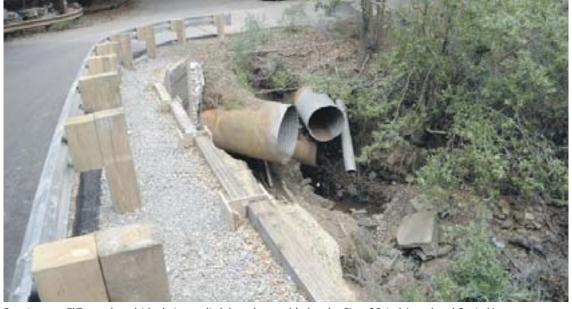
Repairs to an El Toyonal roadside drainage ditch have been added to the City of Orinda's updated Capital Improvement Plan for 2012-2013. Note the aging corrugated metal pipe (CMP). Estimated price tag: \$30,000.
