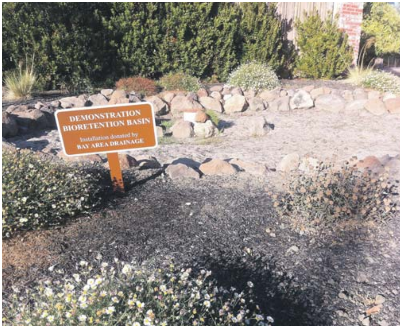
The bio-retention basin in front of 331 Rheem Blvd in Moraga
