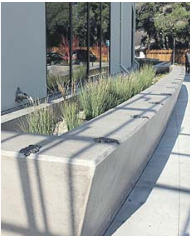
Water collecting planter at the Walnut Creek Library
