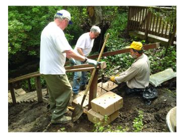
Members of the Kiwanis Club of Moraga replaced the steps that lead down to the stream at the Hacienda de las Flores. New masonry steps next to the La Sala building replace rotting railroad ties that were installed by other Kiwanians a number of years ago. The handrails built then are in good condition and are being retained, according to Sam Sperry, chairman of the project for Kiwanis.
