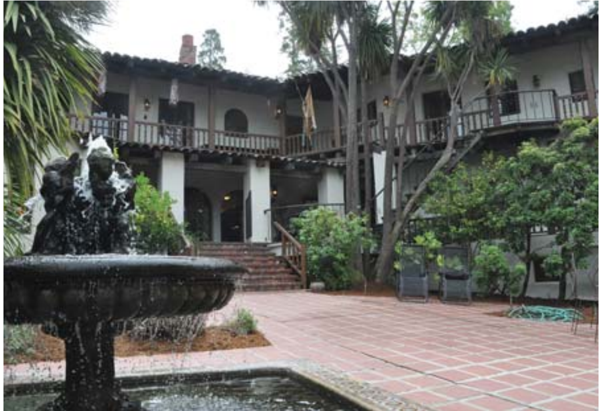
Rear courtyard area with fountain.
