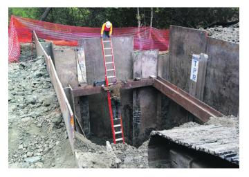
A repair crew is now working its way down to fix a failed drainage system in the Tarabrook neighborhood, which spawned a massive sinkhole last December. A new, sturdier 36-inch concrete drainage pipe will be lowered into this jacking and boring pit - a challenging 25 feet below ground - before workers tunnel and inch the pipe to its final destination. Photo Chuck Swanson
