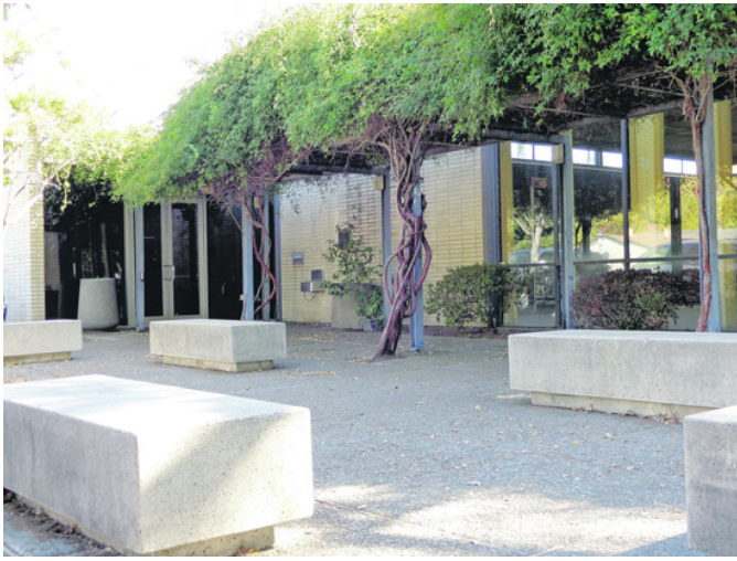
Old library building Photos Cathy Tyson
