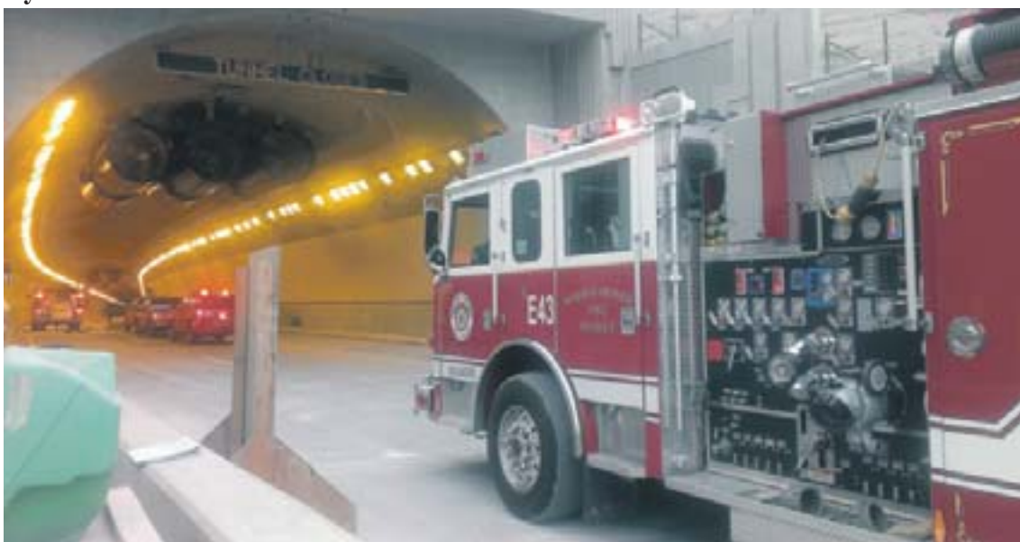
MOFD fire engine at the new bore entrance
