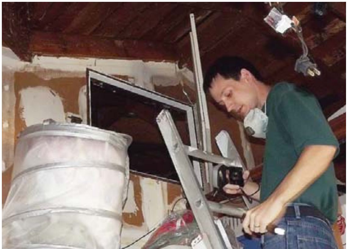
Kyle Bosworth of Eco Performance Builders inspects the Penneys' home.
