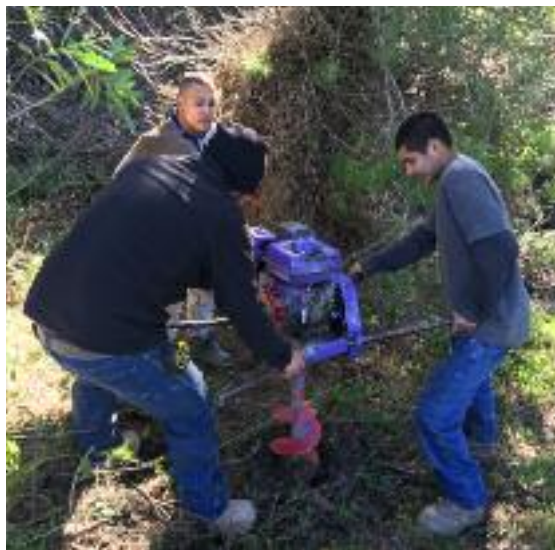
A crew with a post hole digger.
