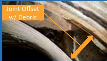
Figure 8: Joint Offset with Debris Intrusion 4/27/16
