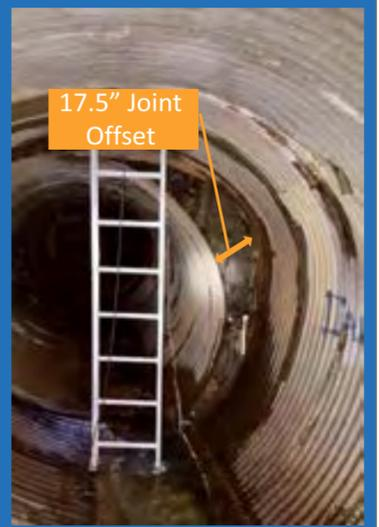
Figure 9: Joint Offset of CMP at Sinkhole Location
