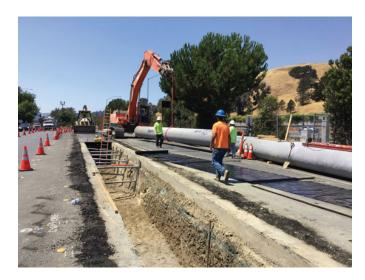
A 30-inch pipe is currently being installed on. Mt. Diablo Boulevard. Photos courtesy EBMUD
