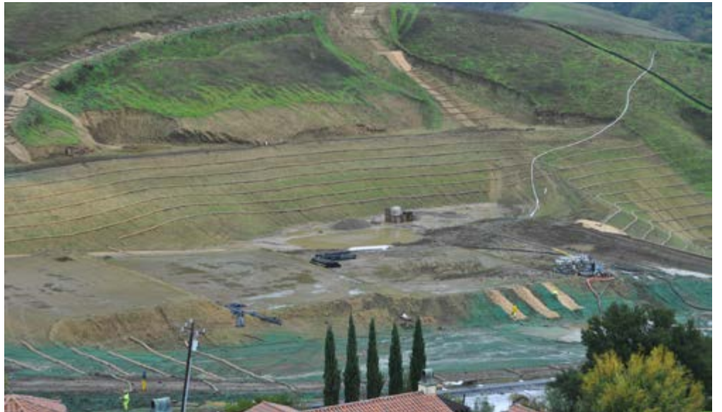
A landslide is slowing work at Bellavista.
