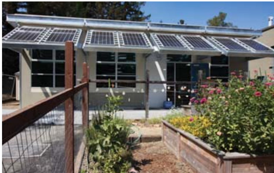
One of several environmentally-friendly Gen7 modular buildings placed on Orinda Union School District campuses this summer. Photo Sora O'Doherty
