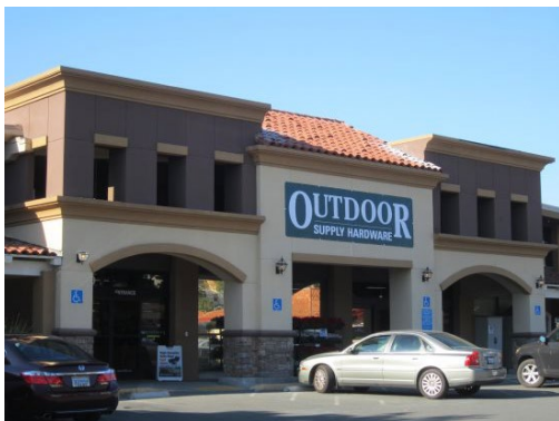
Temporary OSH banner signals "open for business" Photo Vera Kochan
