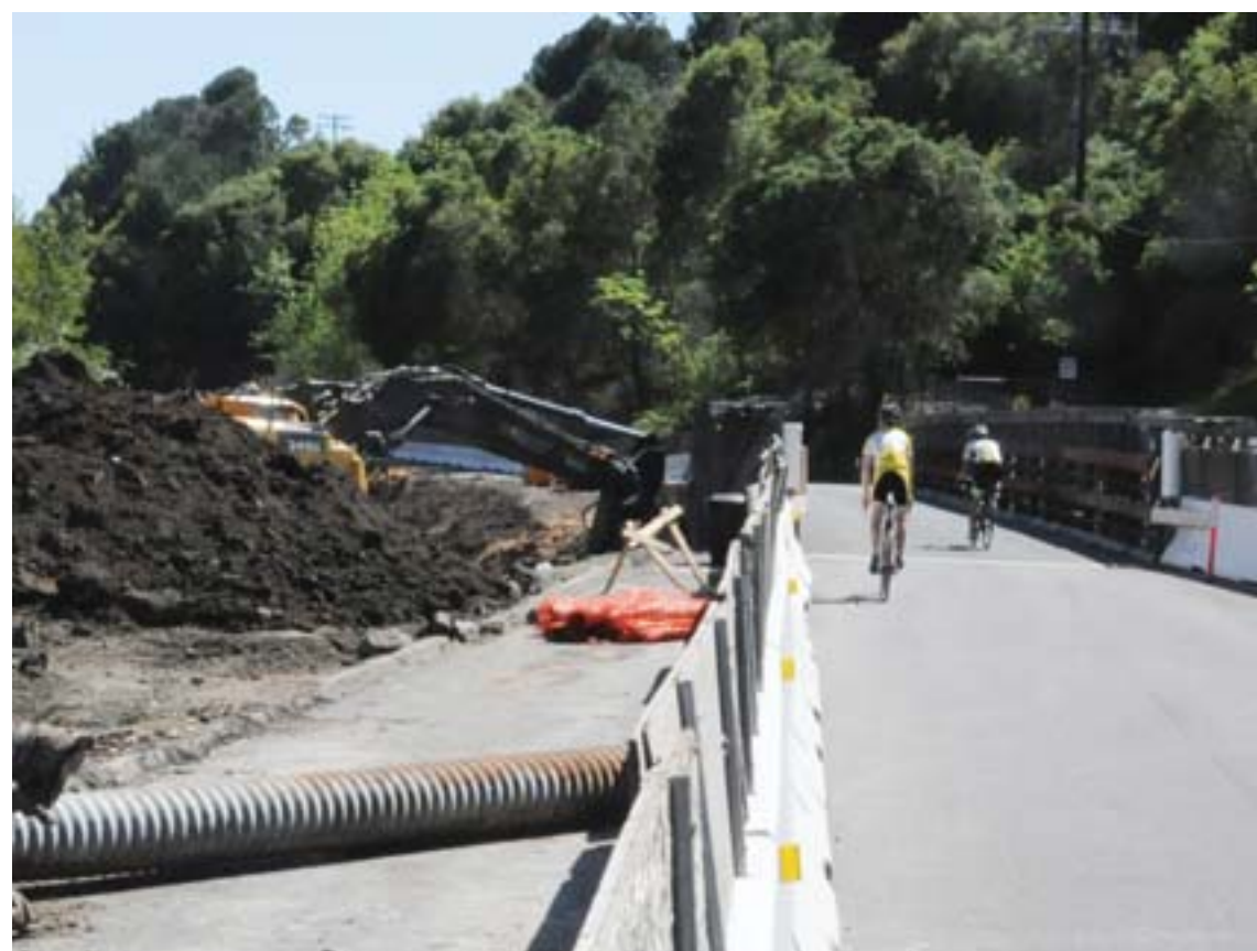
Canyon Bridge work
