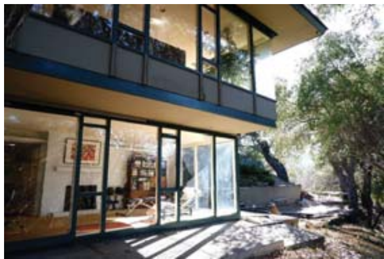
Fully glazed window walls at the southwest corner, looking southeast.
