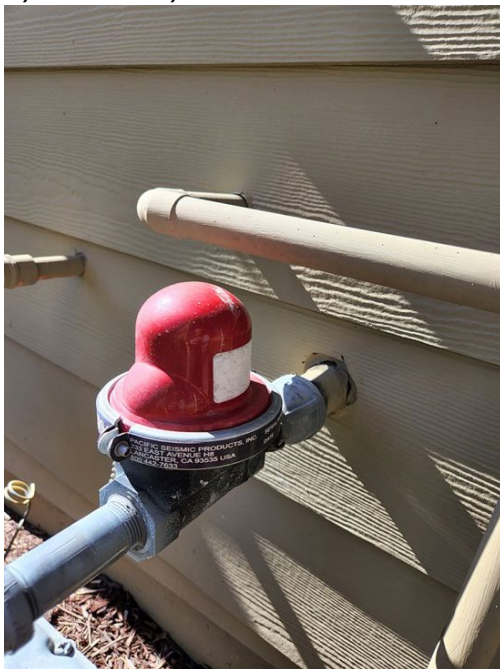
Seismic auto-shutoff valve
