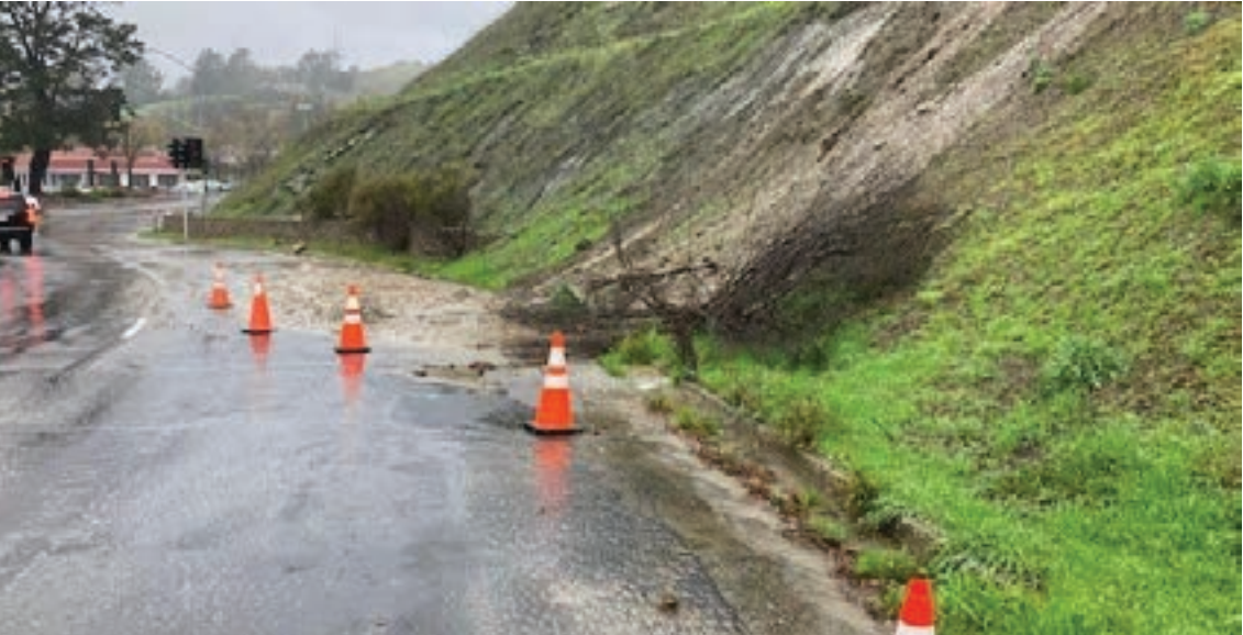
Landslides - Painted Rock debris fell onto Rheem Boulevard
